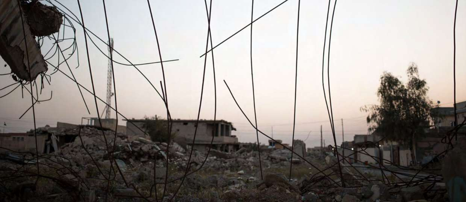
A house in Sinjar city totally destroyed during the fighting in 2017. In some buildings, unexploded rockets and booby-traps remain. © F.Vergnes / HI
