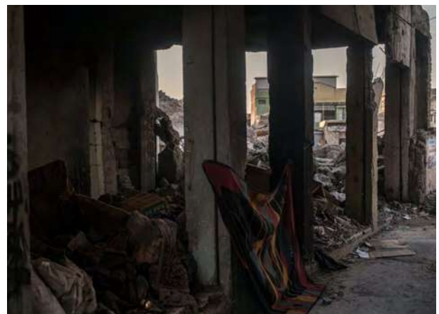
A damaged building contaminated by unexploded rockets serves as makeshift accommodation for its owner. © F.Vergnes / HI
