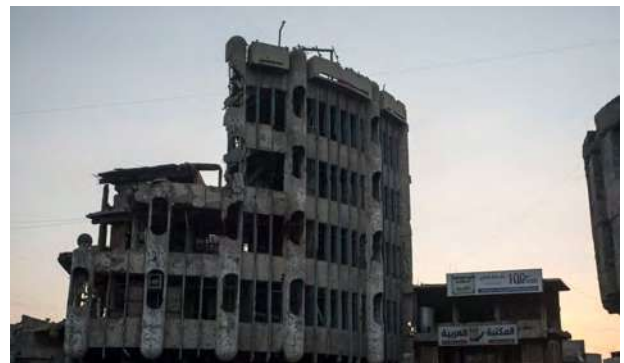
Old apartments and shops destroyed by the intense fighting that took place in Mosul from 2014 to 2017. © F.Vergnes / HI
